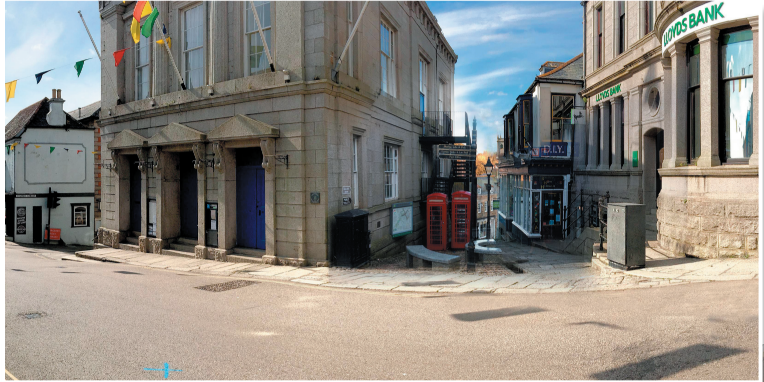
The Guildhall and Market Place existing.
