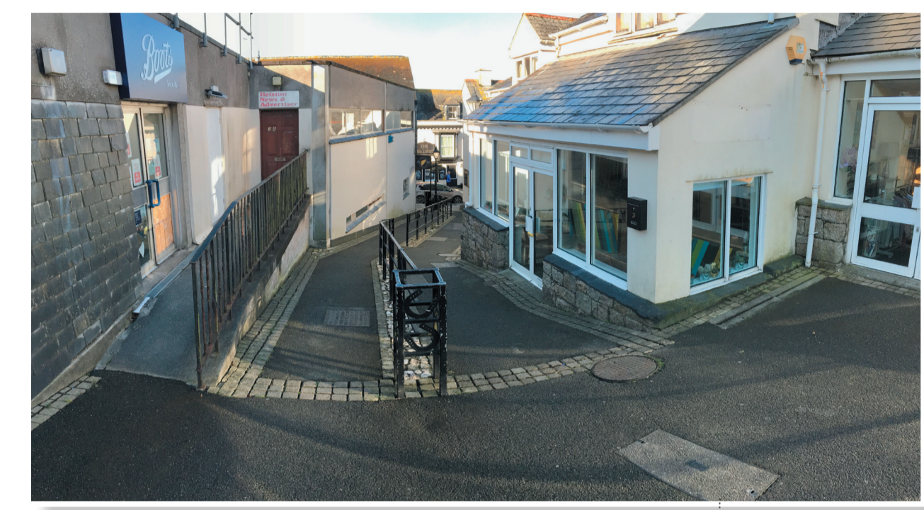
Existing view looking down Horse and Jockey Lane
